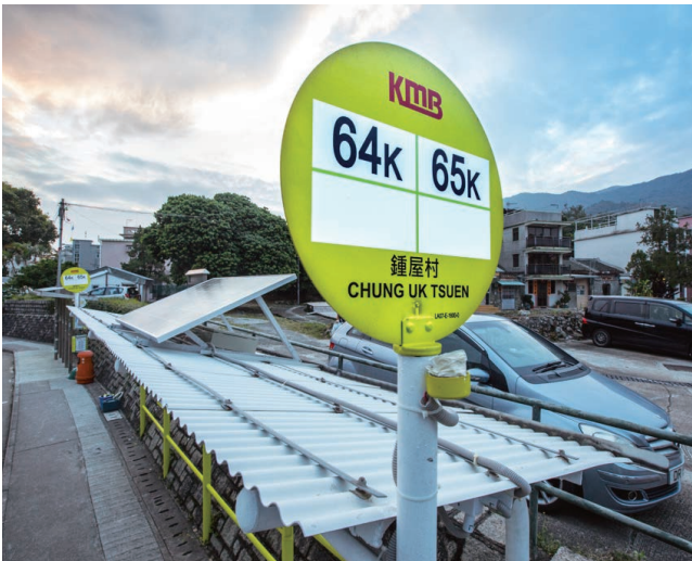
KMB has installed solar panels on the rooftops of bus shelters without an electricity supply 九巴為沒有電力供應的巴士候車亭安裝太陽能供電裝置
